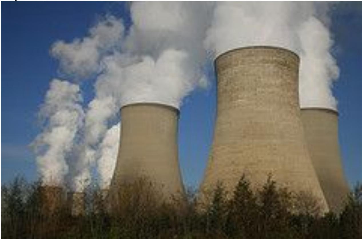
In the UK 90% of electricity generation comes from thermoelectric power stations. Cooling of thermoelectric plants is often achieved by water abstractions from the natural environment. In England and Wales, the electricity sector is responsible for approximately half of all water abstractions and 40% of non-tidal surface water abstractions.
