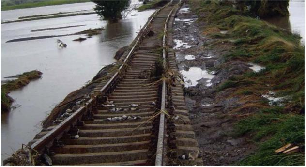
Erosion of the bank of a railway track by heavy precipitation (photo: Wilfried ten Brinke)
